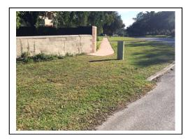
• The sidewalk network suffers from poor transitions at intersections. In several locations along SR 19, sidewalks stop at the apparent property line leaving a grass area between the sidewalk and paved street area. This condition creates a limitation for pedestrians and may be a violation of handicapped accessibility requirements. This condition should be
